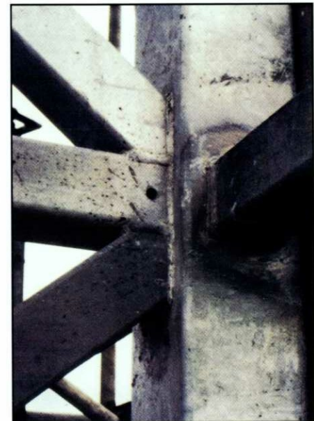
Figure 4: Repair to a weld using a zinc alloy stick.
