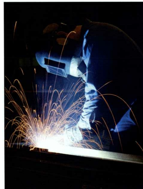
Figure 3: A common cause of coating damage is welding.
