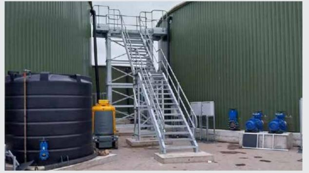
yndhurst Precision was tasked to create two large cat ladders, as well as a stairwell with a landing platform to allow access to two wastewater treatment tanks. Measuring up to seven metres tall, Manchester Galvanizing were called upon thanks to their large hotdip tanks which could safely and appropriately administer the finish of choice.
