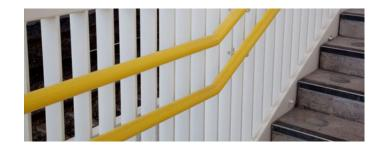
While most standard paints are intended for use on ferrous metals, **Galvacoat**® has been designed exclusively for use on non-ferrous metals, and can be applied in a single coating - without the need for special etch primers. It adheres firmly to the to the galvanized surface and does not allow any salts to form, thus maximising and adhesion and delivering a quality coating that can be typically expected to last up to 15 years.
